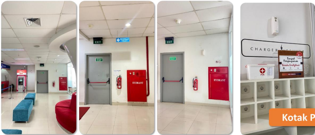
APAR, Hydrant, Emergency Exit
